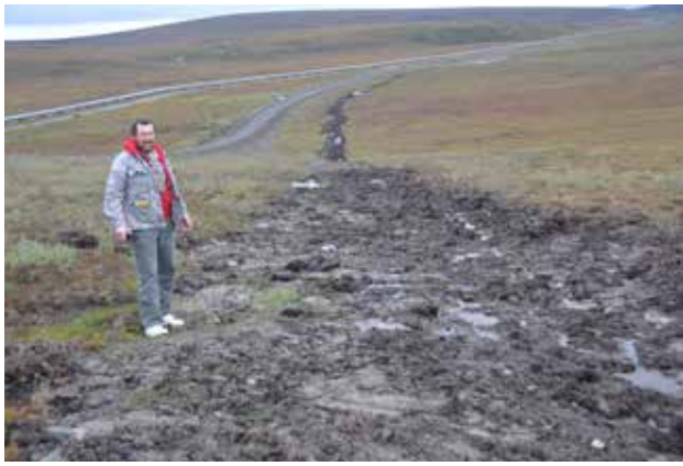
Figure 3.20. Severe tundra disturbance caused by placement of the Quintillion fiber optic cable in summer, near Milepost 305 of the Dalton Highway, 16 August 2016. The width of the damaged tundra in sections constructed in summer is approximately 8.5 m. Photo: DSC 9199.
