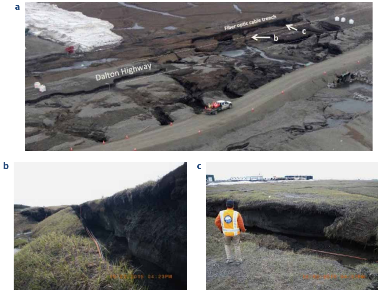
Figure 3.22 (a) Washed out section of the Dalton Highway near the Deadhorse Airport caused by the 2015 Sagavanirktok River flood. Floodwaters threatened the Deadhorse Airport runway (beyond the upper margin of the photo), and the highway acted as a dam preventing water from flowing away from the airport toward the Sagavanirktok River (lower right). When the road was breached to allow floodwaters to drain away from the airport, massive erosion of ice wedges occurred between the Quintillion fiber optic cable trench and the river. Approximate locations and directions of the photos in (b) and (c) are shown by the white arrows in photograph (a). Orange fiber optic cables are visible in all three frames. Photos courtesy of AK Department of Transportation & Public Facilities.
