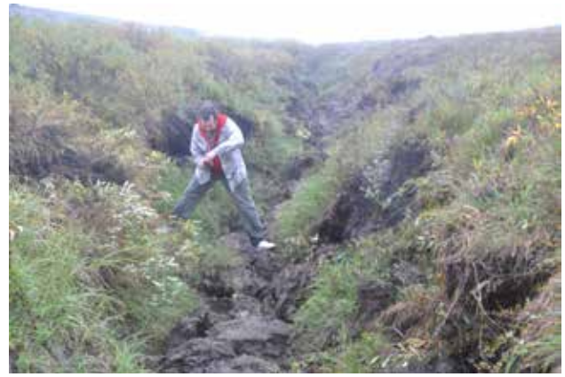
Figure 3.21. Thermokarst in the trench of the Quintillion fiber optic cable, Sagwon Upland, near Milepost 355 of the Dalton Highway, 16 August 2016. Photo: DSC 9275.
