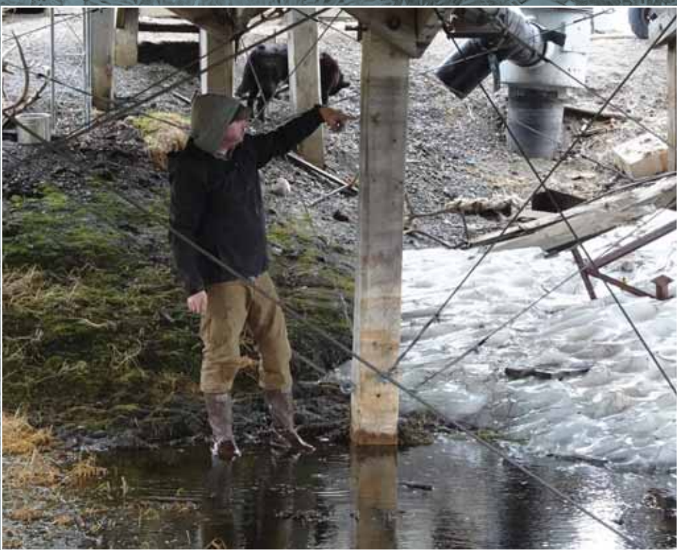
Most piling beneath village housing was originally embedded 10 feet (~3 m). It appears that those piles embedded in ice wedges have as little as 1 m of embedment remaining due to ground subsidence.
