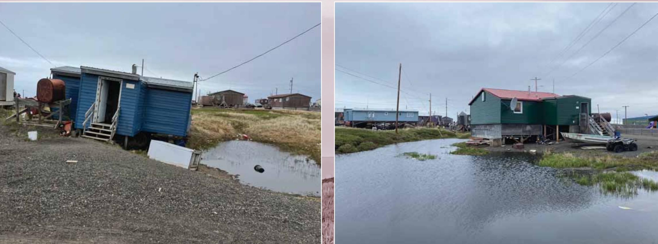
Ground subsidence of up to 3 meters has destabilized homes, utility poles, and fire hydrants, and caused frequent breaks in underground water and sewer lines, resulting in multiple health and safety risks. Deep cracks in the terrain, sinkholes and surface water ponding create hazards for tundra travel and for children playing outdoors. These photos show the impacts of ice-wedge thermokarst on two homes. A 2022 survey by the Cold Climate Housing Research Center found about two-thirds of homes with damage due to thaw settlement and 70% affected by ponding.
