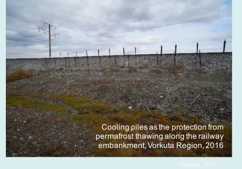
This problem leads to high costs for the regular repair or construction of protective systems, such as cooling pipes.
